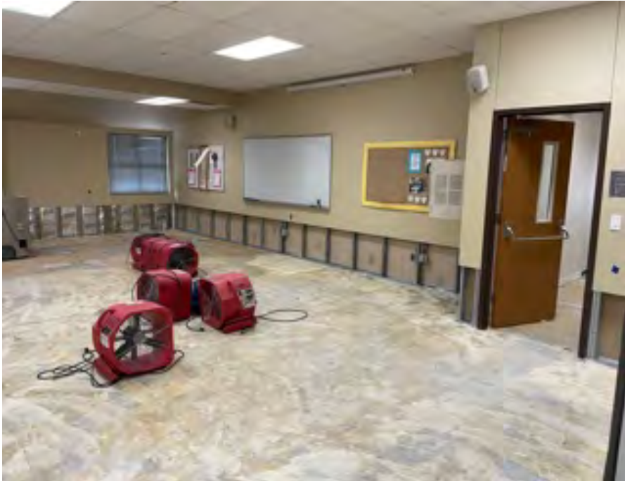
Floor fans drying out PACE classroom after removal of carpet
